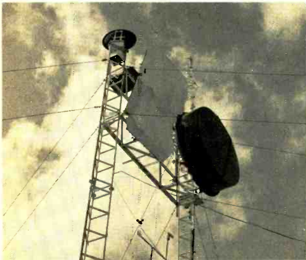
WTVJ Microwave master pick-up and transmission system loop atop station.
